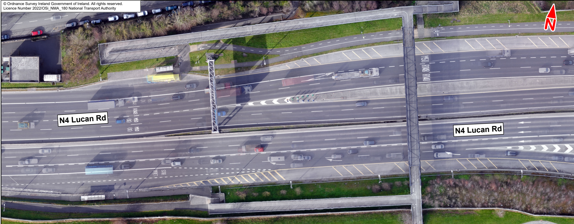
A) N4 LUCAN ROAD/M50 JUNCTION 7
