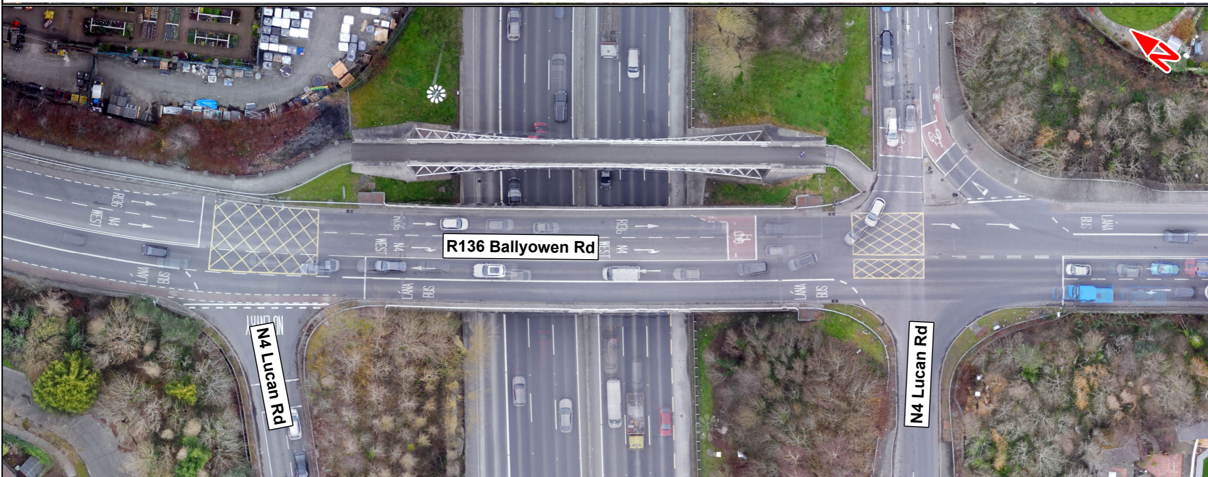
B) N4 EB ON-SLIP / WB OFF-SLIP / BALLYOWEN ROAD
