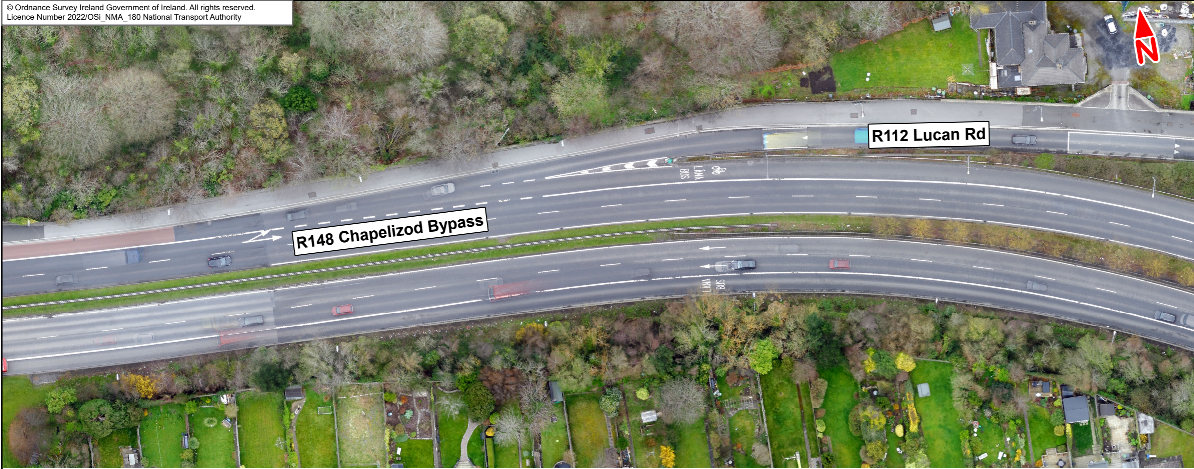
A) R148 CHAPELIZOD BYPASS/R112 LUCAN ROAD JUNCTION
